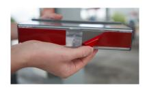
3. Install the MDU on the top, left-hand side of the dispenser next to the inner white riser—one (1) MDU per each fueling position on the dispenser.
